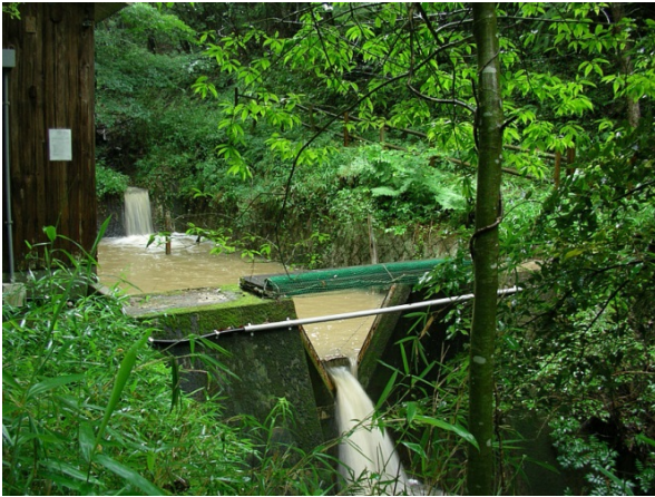
出水時の量水堰堤 The gauging weir at a storm event
