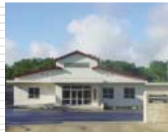
庁舎 Office building
