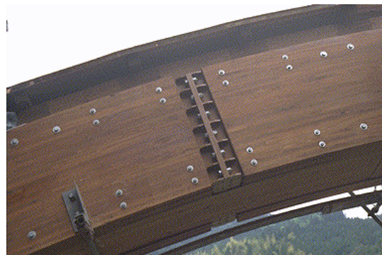
Close up of Box Arch Beam Joint 接合部近影
