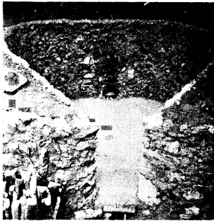
4. かま底窯壁の仕上 Phot. 32 Completion of kiln bottom
