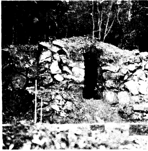
1. 古がまとりこわし Phot. 29 Pulling down of old kiln
