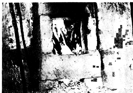
8. 口 焚 状 況 Phot. 8 Pre-heating in kiln inlet
