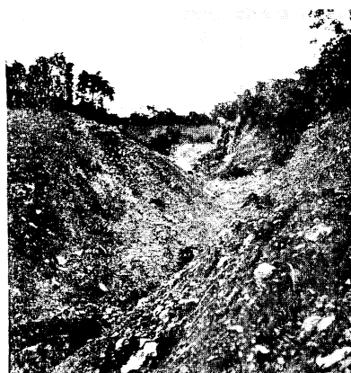
写真 2 土層と岩盤の接触不連続による崩壊 (稲積川) Phot. 2 Landslide due to discontinuous plane between upper soil layer and bed rock.
