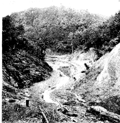
Phot. 64 溜池の欠潰 (大正池) Collapse of irrigation pond
