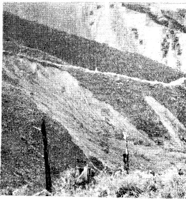
Phot. 3 伐跡地の崩壊 Landslides in cut-over areas
