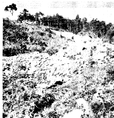
Phot. 65 山腹工事と崩壊 Hillside works and Iandslide
