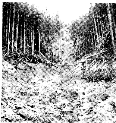
Phot. 11 地氇性崩壊と山津波 (32林班) Landslide of landcreep type and upstream mud and stone flow
