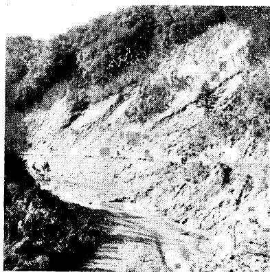
Phot. 55 曲流による溪岸崩壊 Landslide along stream due to meander
