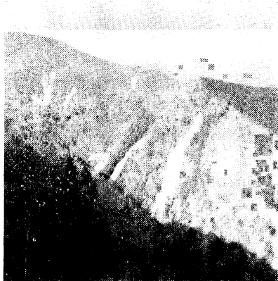
Phot. 47 林地の崩壊 Landslides in forest land
