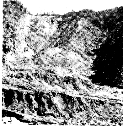
Phot. 43 崩壊と山津波 Landslide and upstream mud and stone flow
