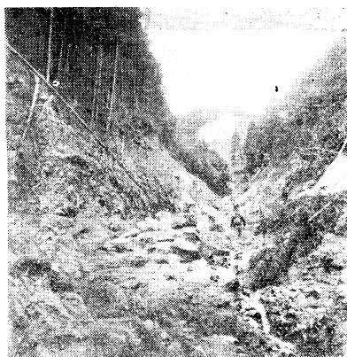
Phot. 13 山津波 (30林班) Upstream mud and stone flow
