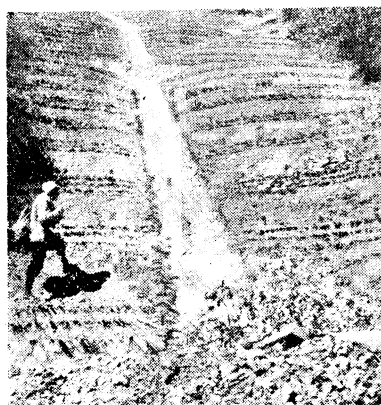
Phot. 59 山腹工事 Hillside works
