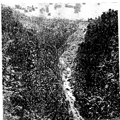
Phot. 50 湧水による山腹滑落 Sliding of soil layers upon bed rock due to welling
