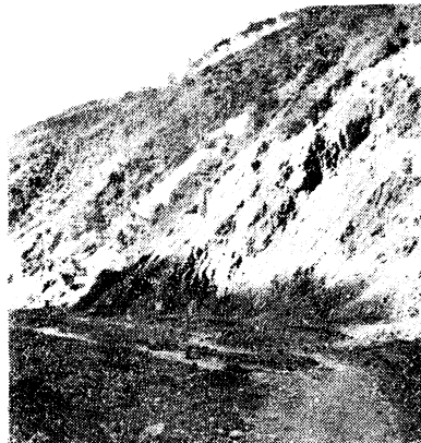
Phot. 69 溪岸崩壊 Landslide along stream
