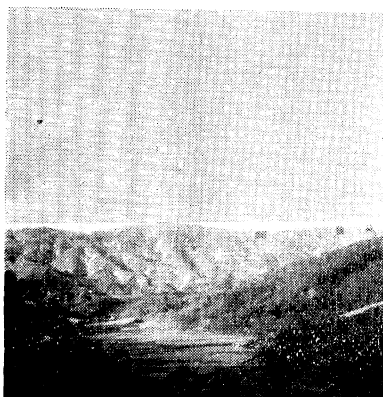
Phot. 78 崩壊地遠望 A distant view of landslides
