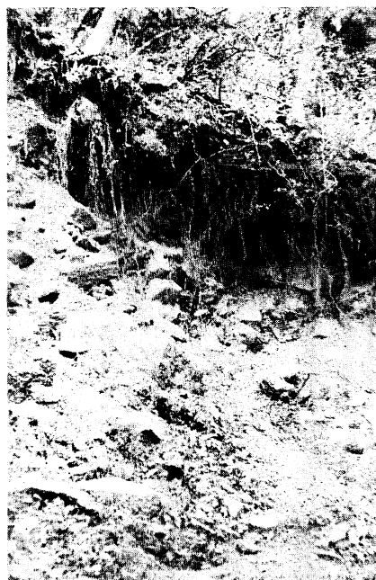
Phot. 8 崩 壊 Landslides.
