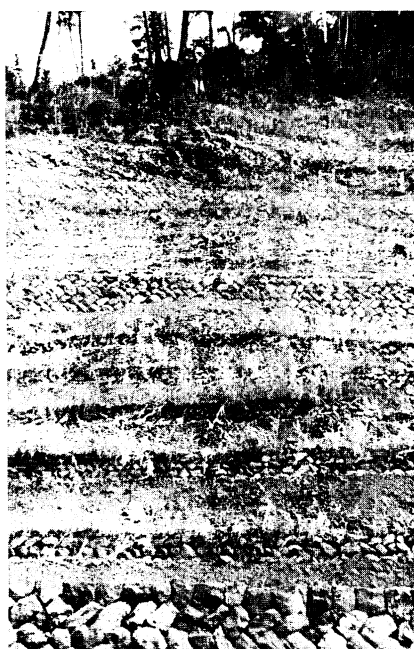
Phot. 12 石筋工 Simple terracing stone works.
