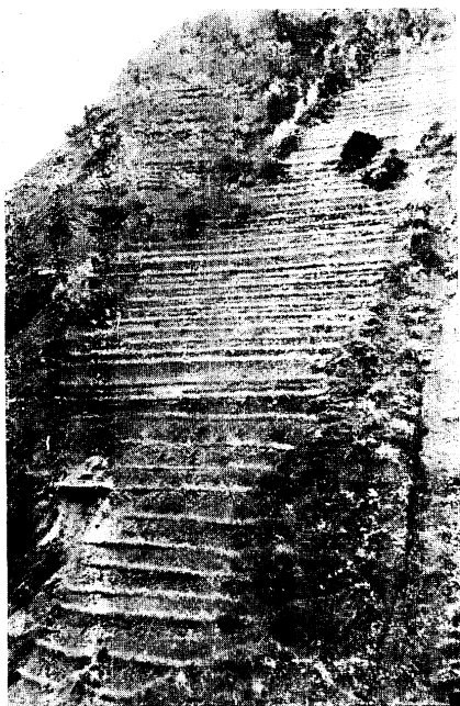
Phot. 25 石礫地の施工 Working at stony area.
