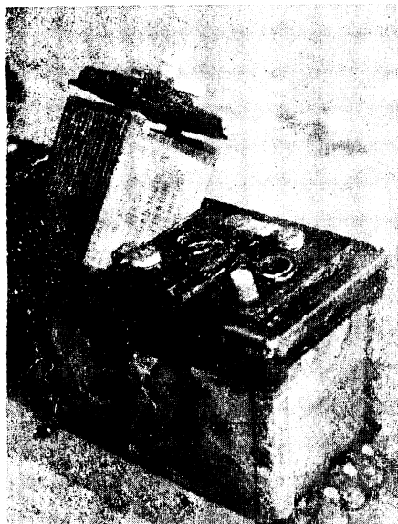
Fig. 16 蓄電池の組み立て Formation of storage battery with wooden separator.
