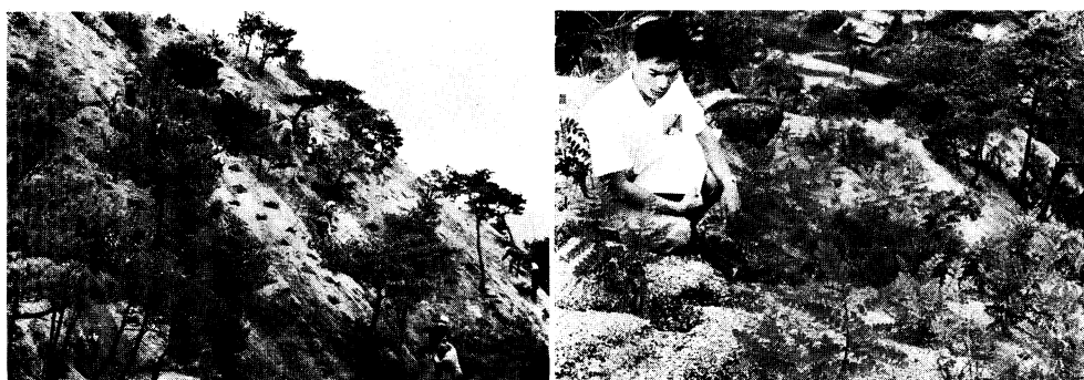
a. 穴掘りと施肥 Digging planting holes and fertilization. b. さし付け後3か月 After 3 months.
