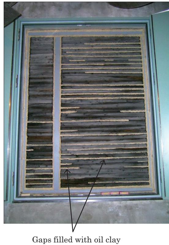
Photo 2 Japanese larch sound barrier of which the gaps allowing light through were filled with oil clay.
