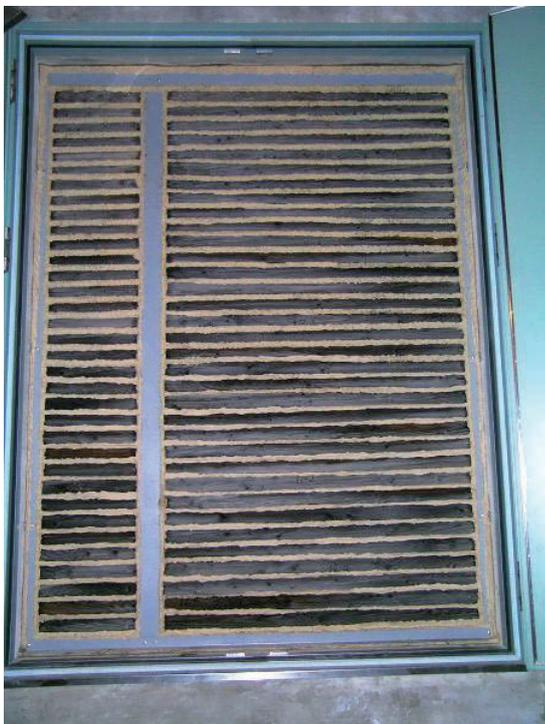
Photo 3 Japanese larch sound barrier, the joints of which were entirely filled with oil clay.
