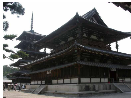
Photo 3. Horyu-ji Temple, oldest wooden structure in the world
